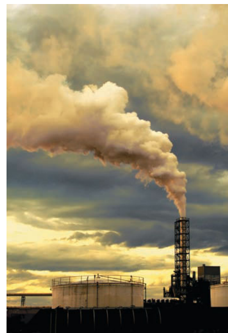
▲ The flow of gases from a smokestack can be measured by releasing ^{41}\text{Ar} and monitoring its passage.
