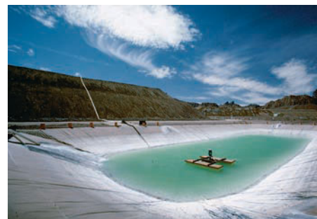
▲ A cyanide leaching pool for extracting gold at the Picacho Gold Mine in the Mohave Desert.
