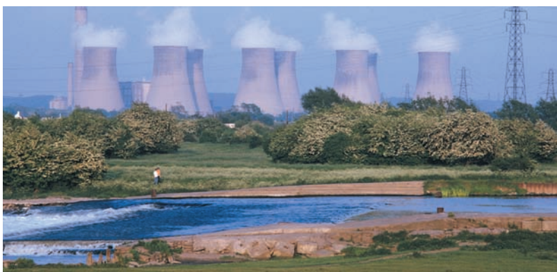
Water is used to absorb heat from nuclear reactors. The water is then cooled in cooling towers before it is returned to the environment.
