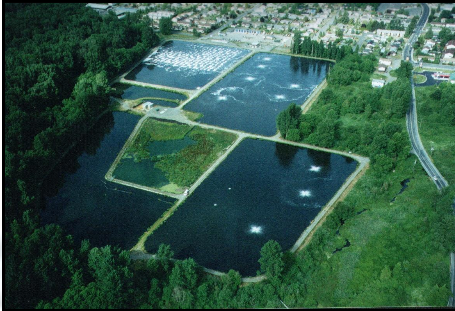
Figure: Sewage lagoons in a wastewater treatment plant
